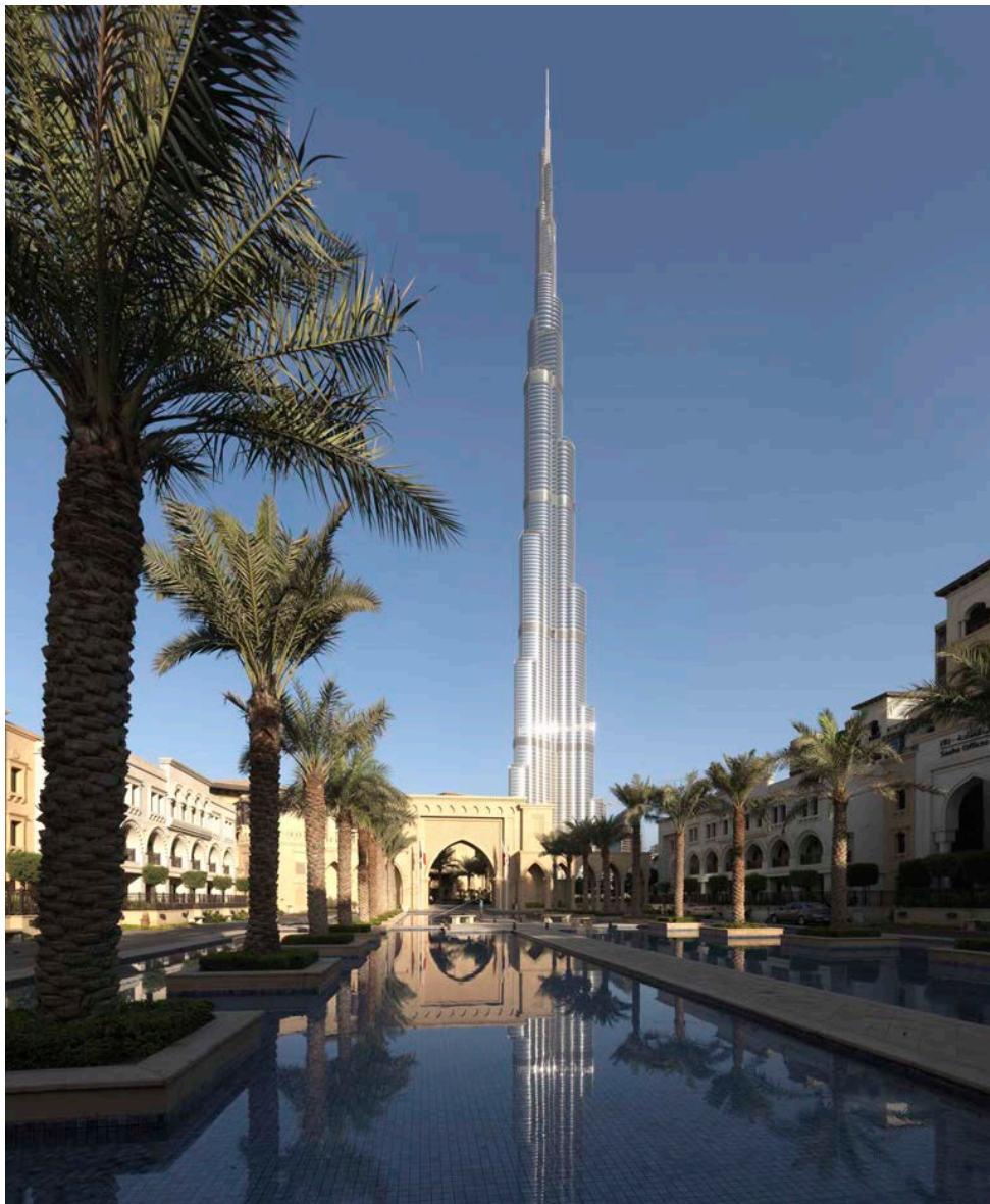
Figure 4: Burj Khalifa, Dubai, the world's tallest building. (Courtesy: Adrian Smith + Gordon Gills Architecture; photograph by J. Steinkamp).
